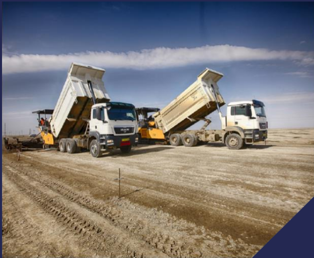
Road Construction & rehabilitation
