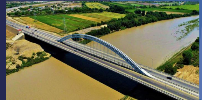
Alat-Astara highway, bridge over Kura river
