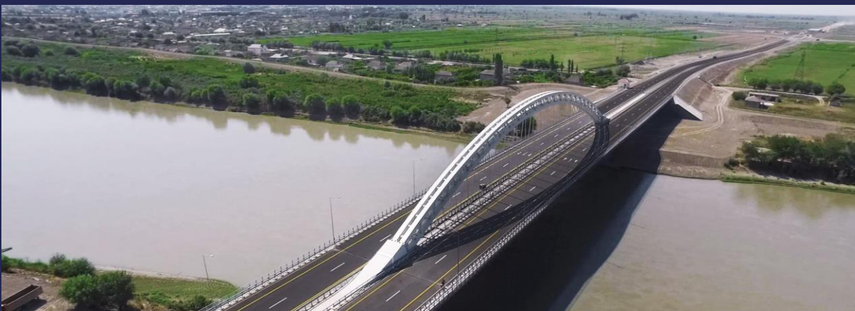
Alat-Astara highway, bridge over Kura river. Length : 362.9 m- Width : 29.8 m- Height above water level – 15 m
