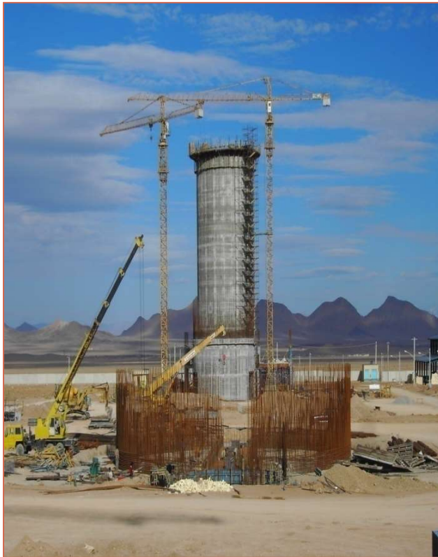
2200ton Sarooj Cement Plant, Execution of silos by Sliding form
