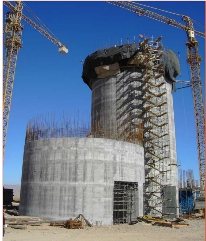
2200ton Sarooj Cement Plant, Execution of silos by Sliding form
