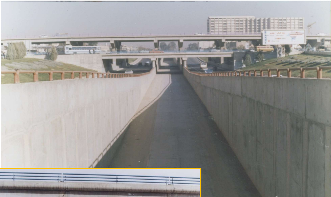
Esfahan Northern Subway Tunnel U-Wall tunnel of part's 5
