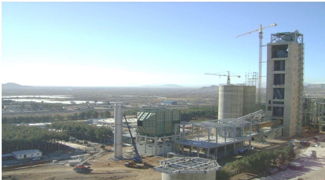
3300ton Sepahan Cement Plant, Execution of cooler grader and steel structures
