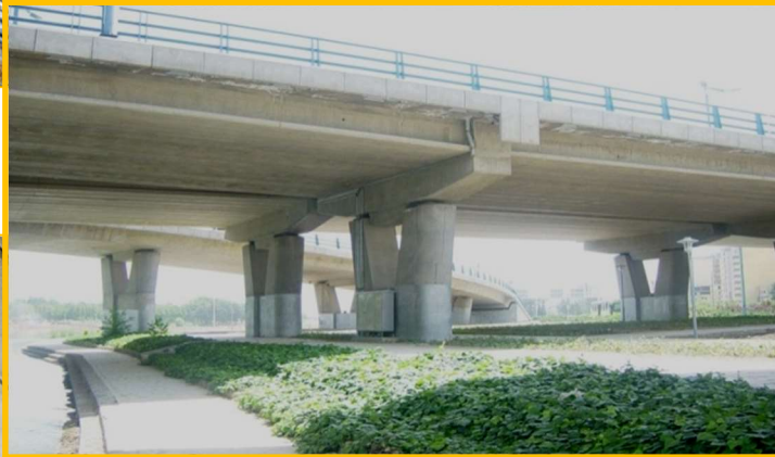
Qadir Bridges complex Precast beams part of view
