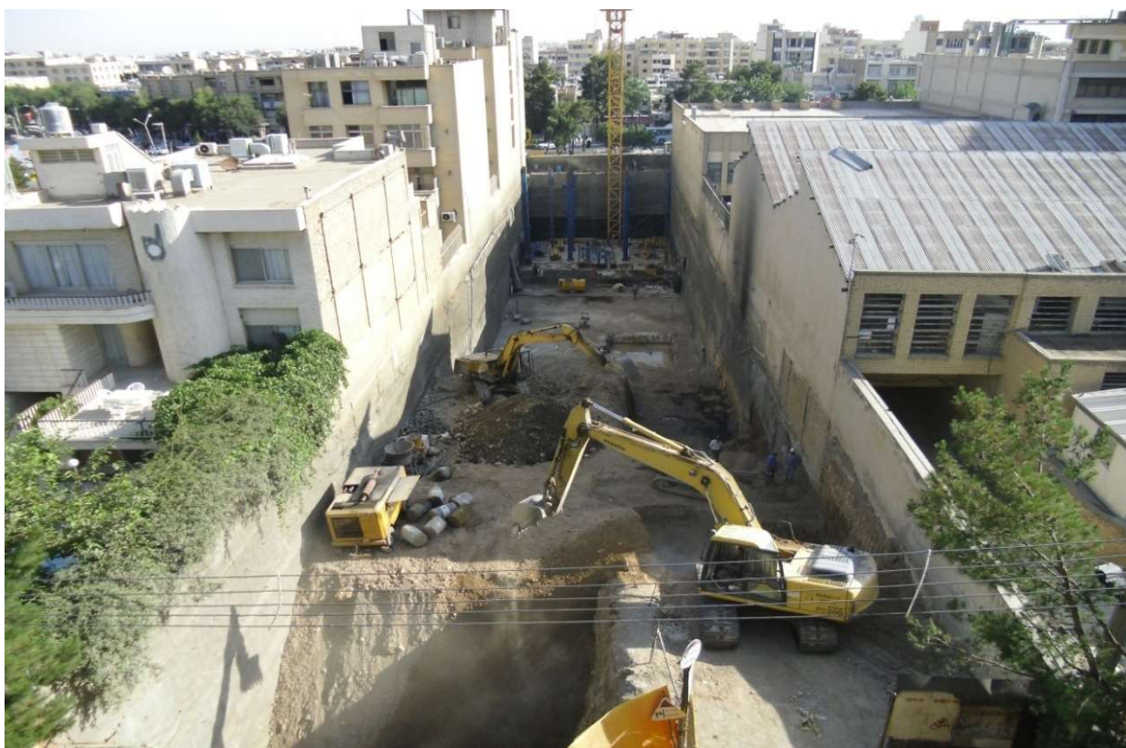
Bank of Tejarat branches management building excavation and nailing
