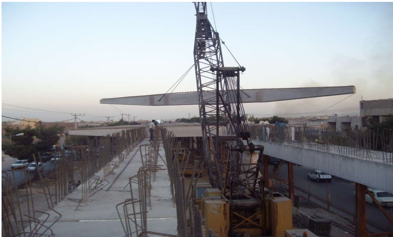
Imam Khomeini highway overpassing bridge, installing transverse girder in a normal traffic day
