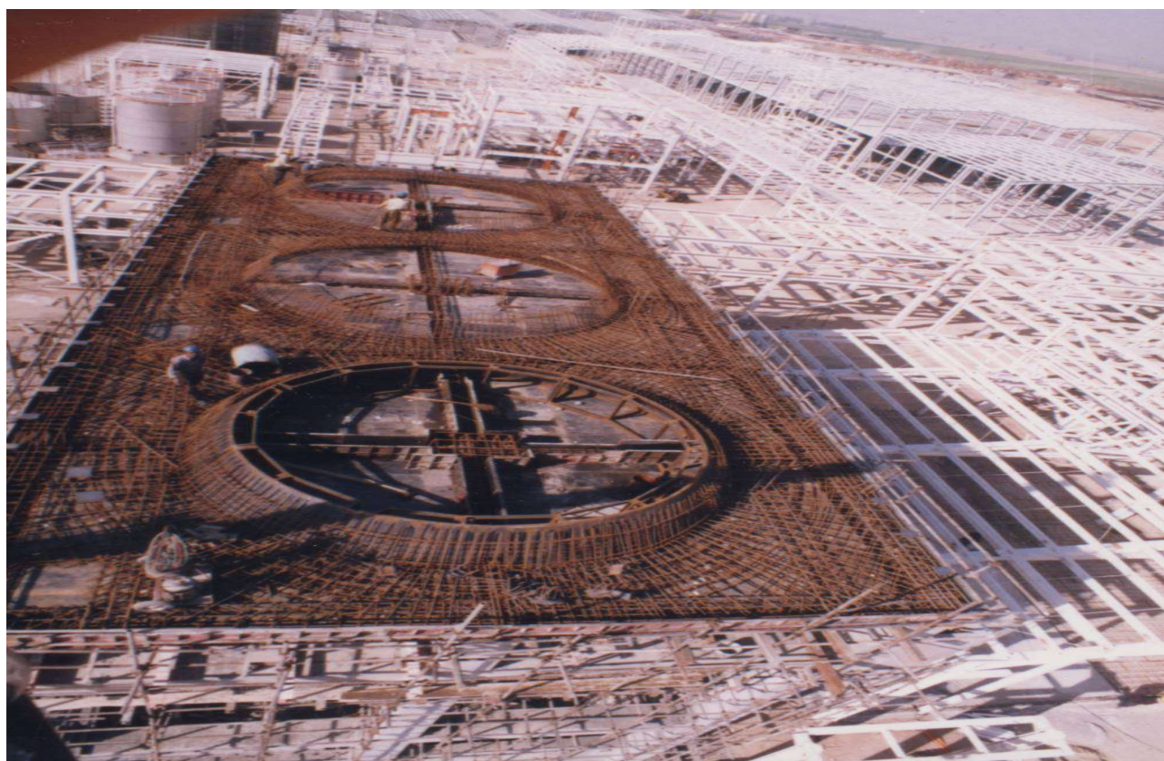
New Polyacryl Plant, Part of Tank Form foundation
