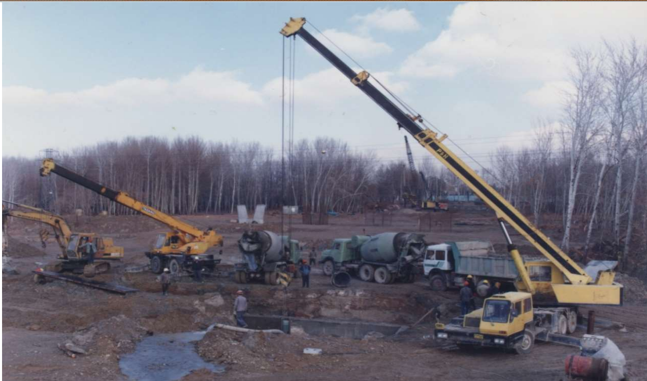
Qadir Bridges complex water draining and concrete filling
