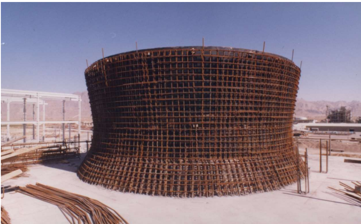
New Polyacryl Plant, Part of Tank Form foundation
