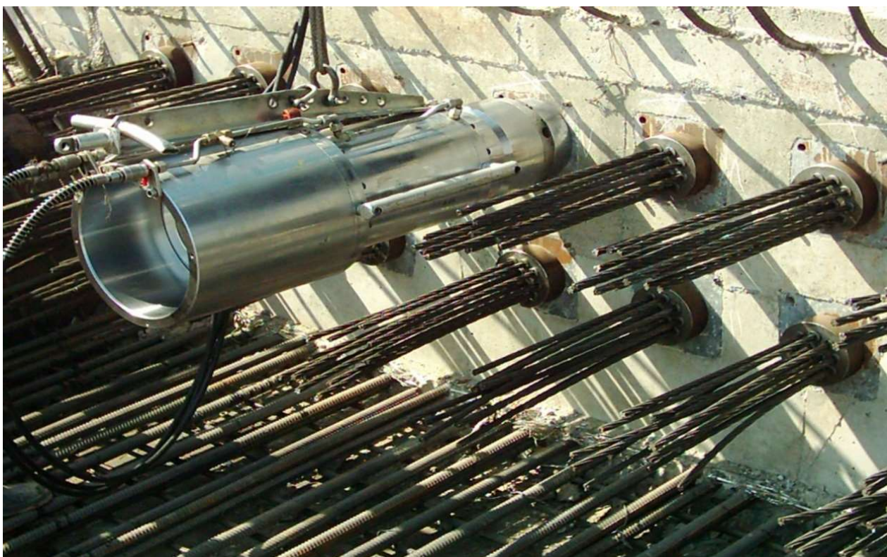
Defea-e-Moqadas Stack Interchange & Flyover, Prestressing No. 100, 200 and 300 bridge Strands
