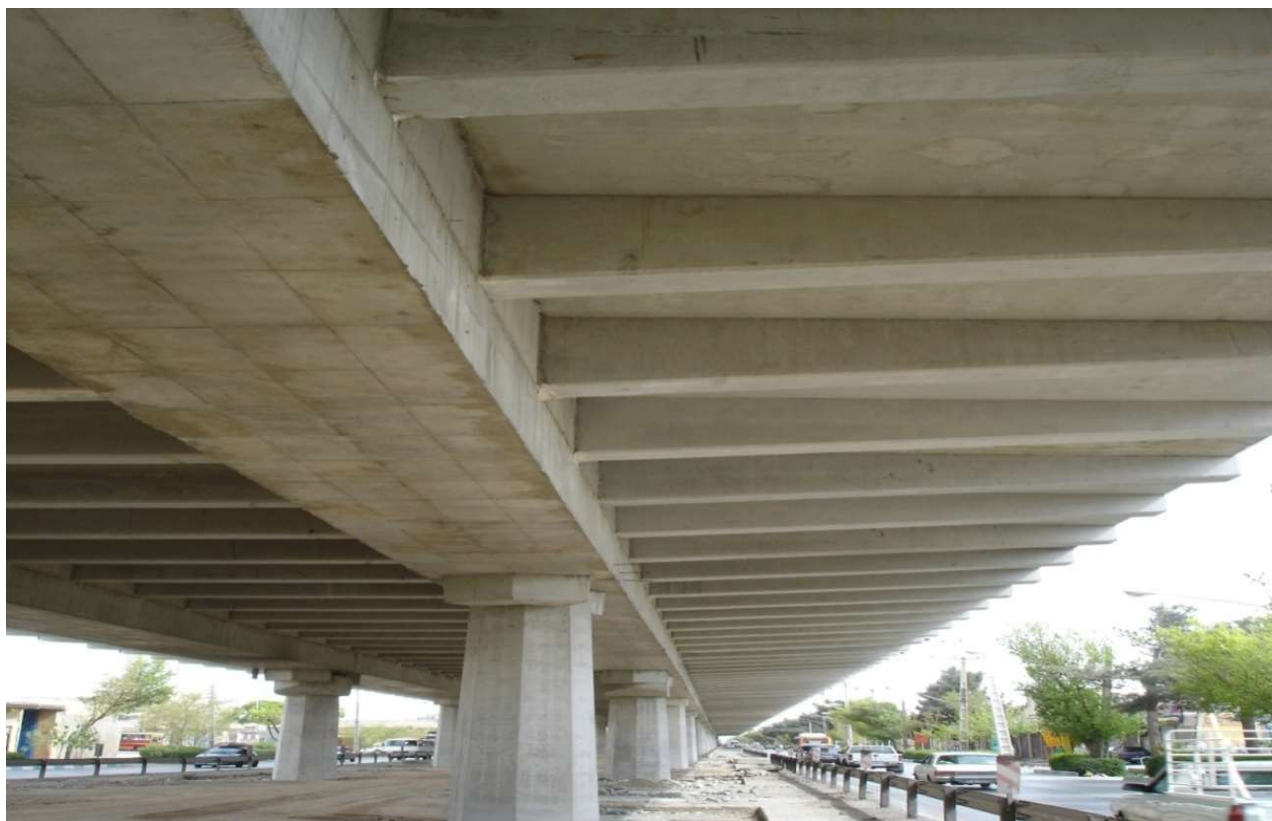
Imam Khomeini highway overpassing bridge, Cantilever beam side view
