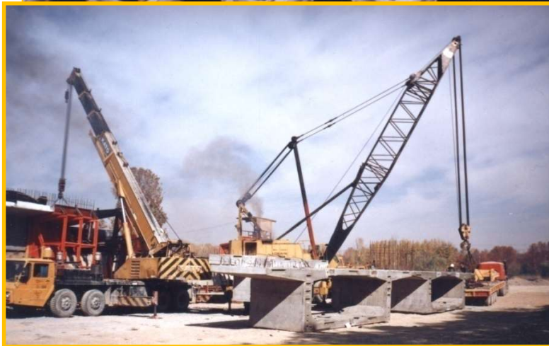
Qadir Bridges complex, Bridge segment, loading and depo-off
