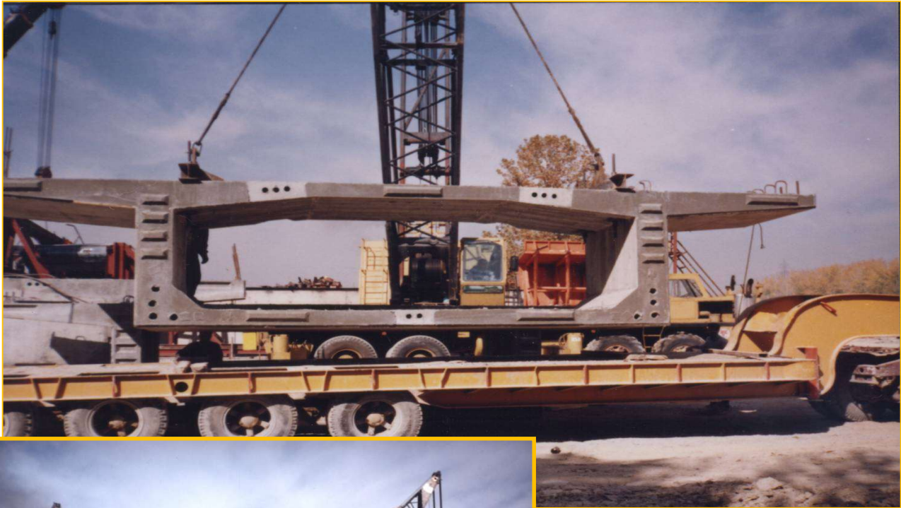
Qadir Bridges complex, Bridge segment, loading and depo-off
