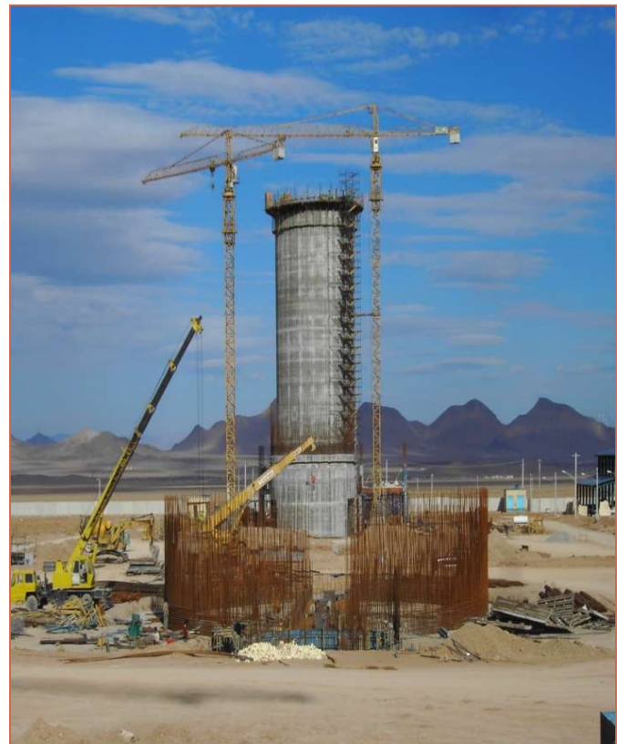
2200ton Sarooj Cement Plant, Execution of silos by Sliding form during a short time
