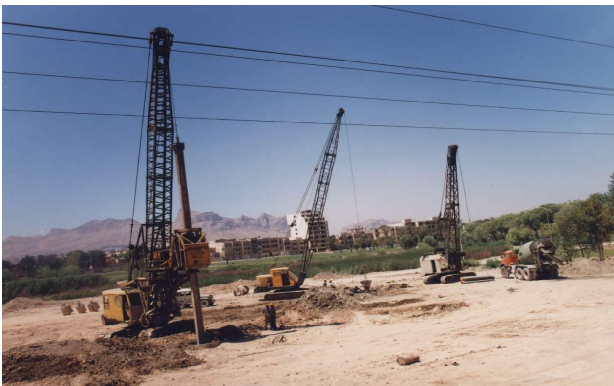
Qadir Bridges complex, Pile foundation
