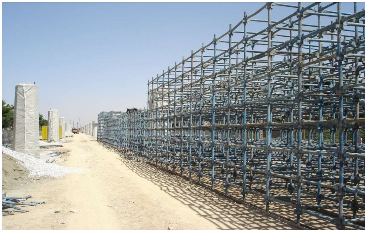
Imam Khomeini highway overpassing bridge, Assembled scaffolding for longitudinal Girders
