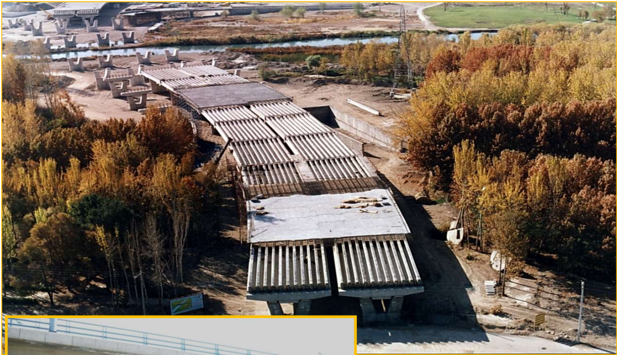
Qadir Bridges complex Precast beams part of view
