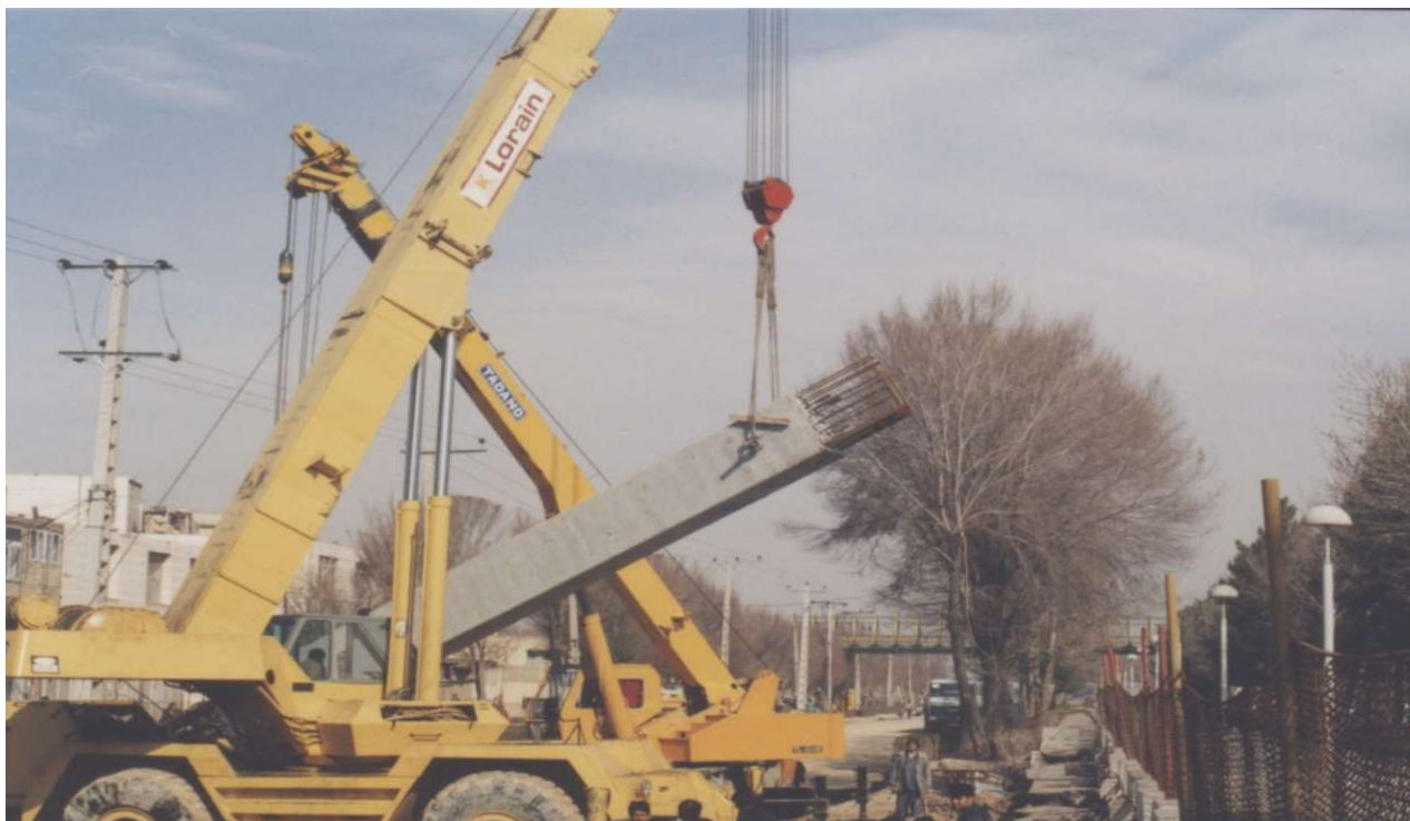
Esfahan Northern Subway Tunnel Erecting Precast piles with 15ton weight and 14m height
