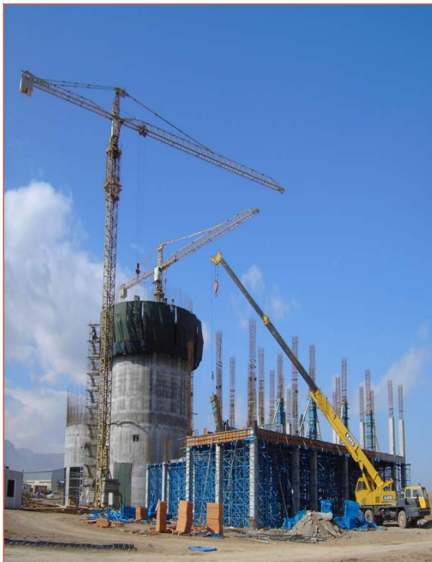
2200ton Sarooj Cement Plant, Execution of silos by Sliding form during a short time
