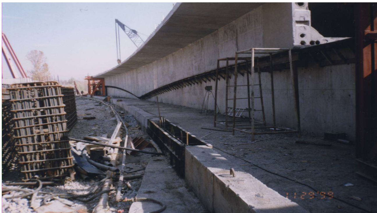
Qadir Bridges complex, Workshop of Precast Segment and sliding Formwork
