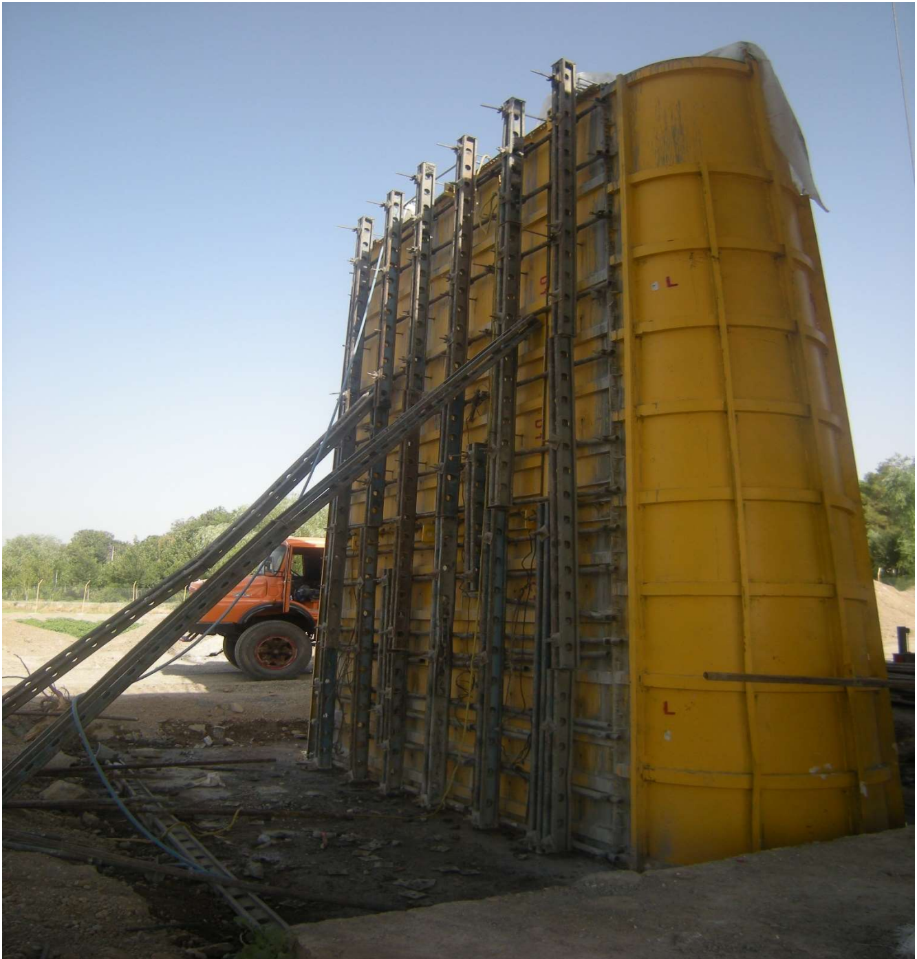
Pol Felezi, Pier Formwork
