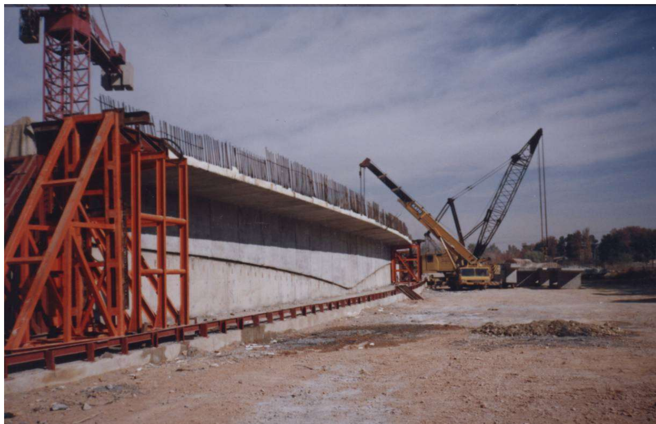
Qadir Bridges complex, Workshop of Precast Segment and sliding Formwork
