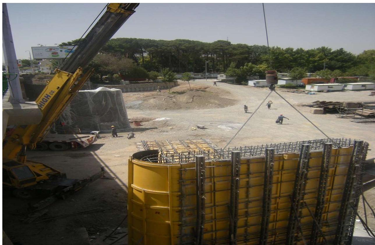
Pol Felezi bridge, Abutment and Piers Formwork
