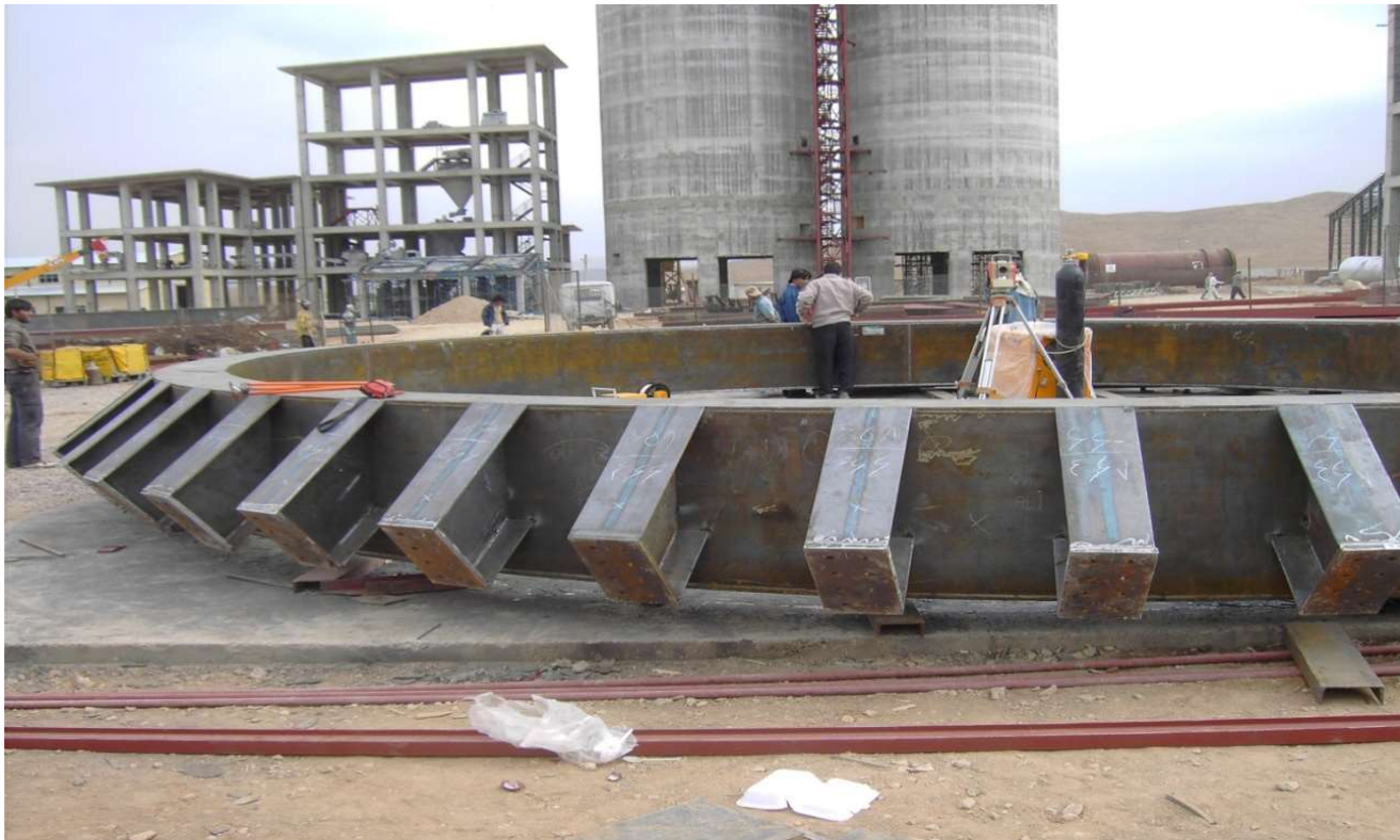
2200ton Sarooj Cement Plant, Ring steel Erection and installed in 40m height
