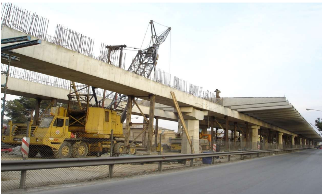
Imam Khomeini highway overpassing bridge, 140ton crane on Erecting Precast Girders
