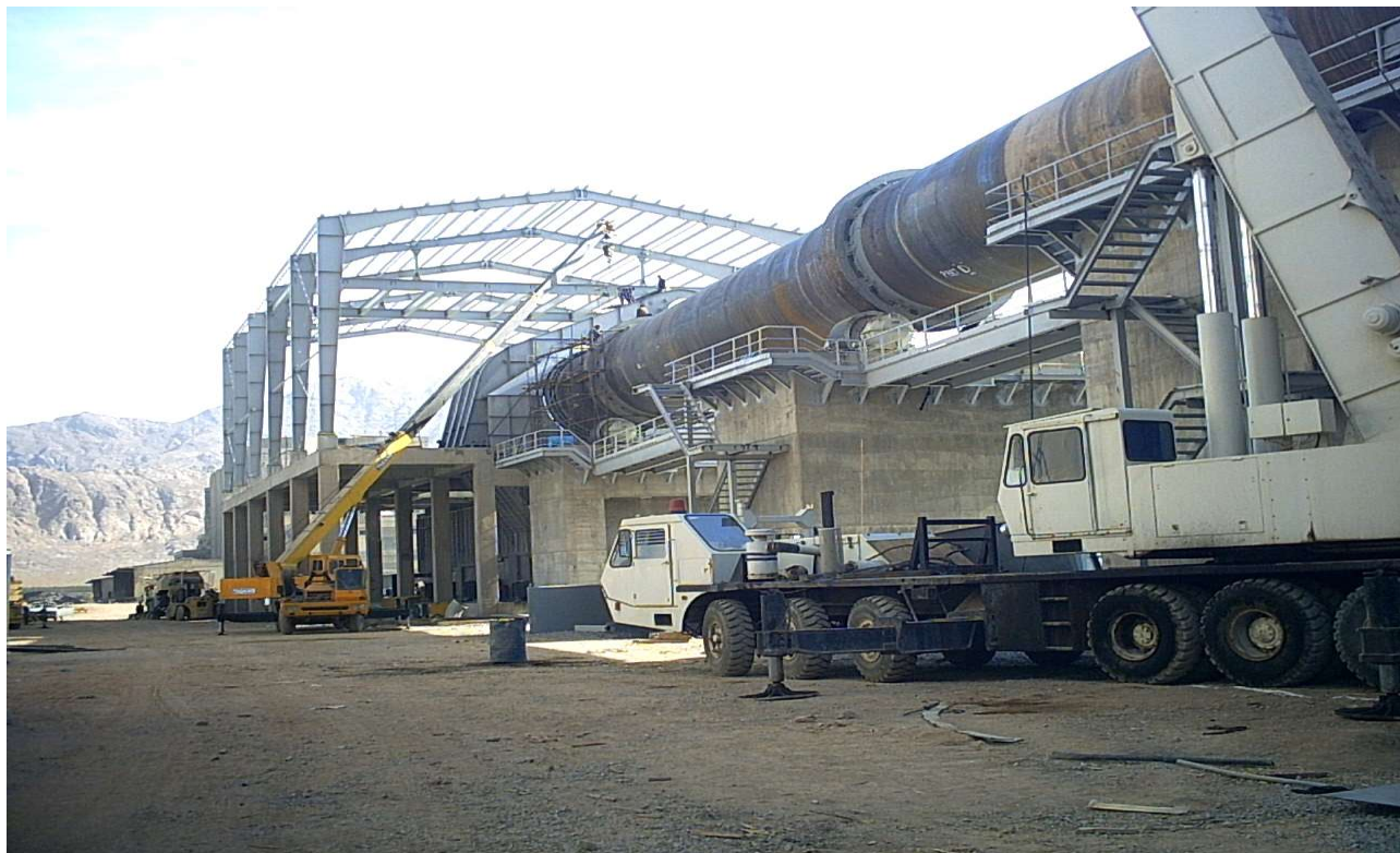
3300ton Sepahan Cement Plant, Cooler Furnace base grade and steel Structures
