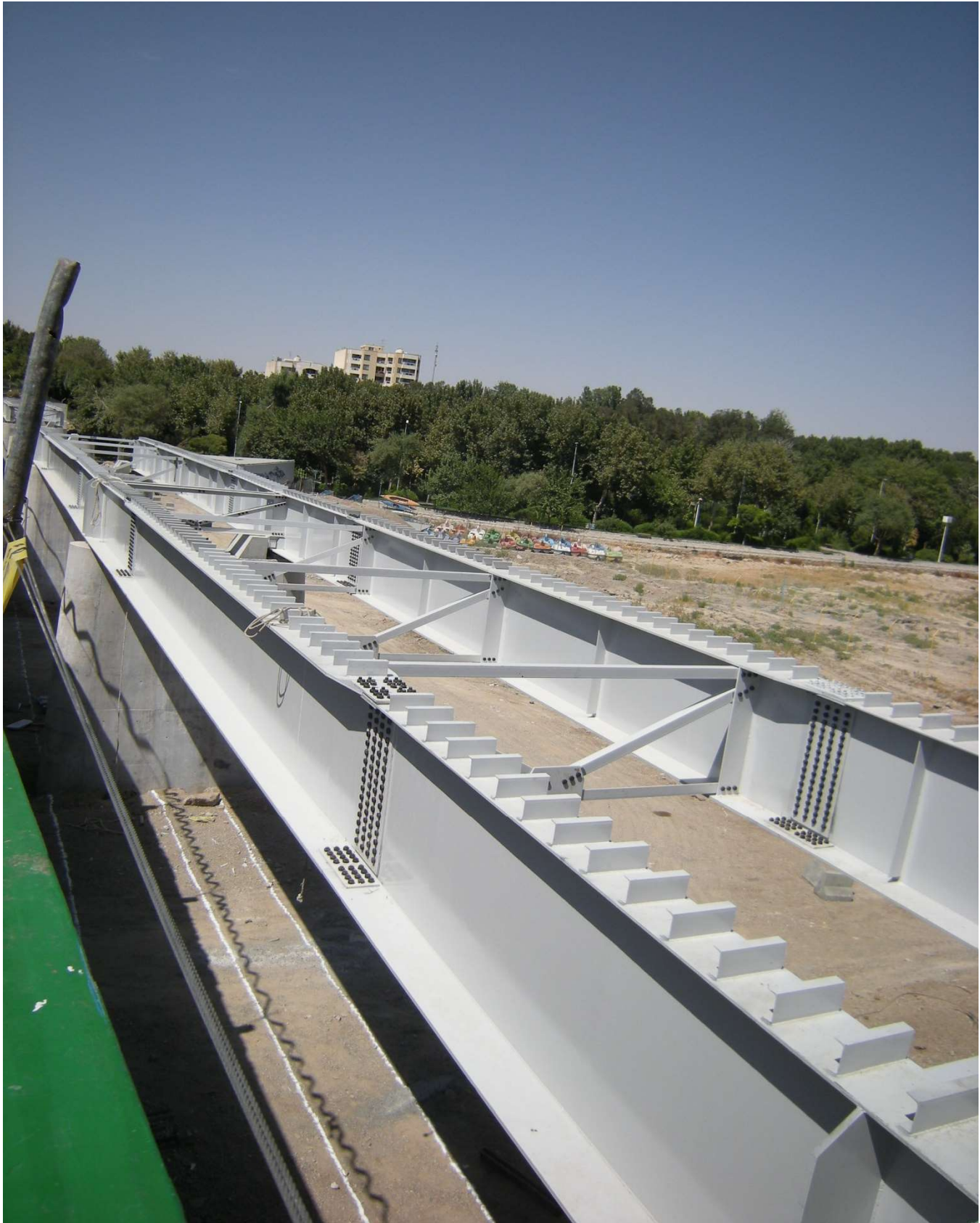
Pol Felezi Bridge, Main Steel Beams
