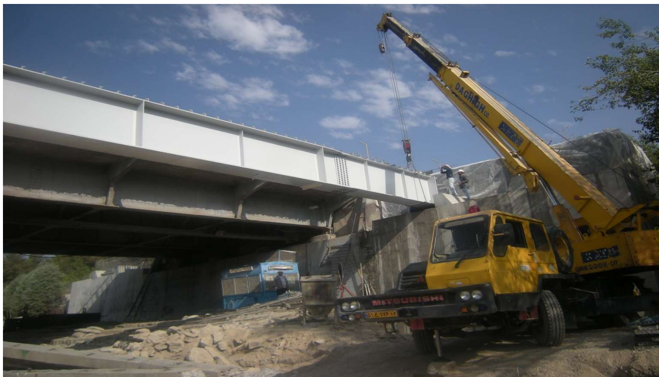
Pol Felezi Bridge, Main steel Beams Installation
