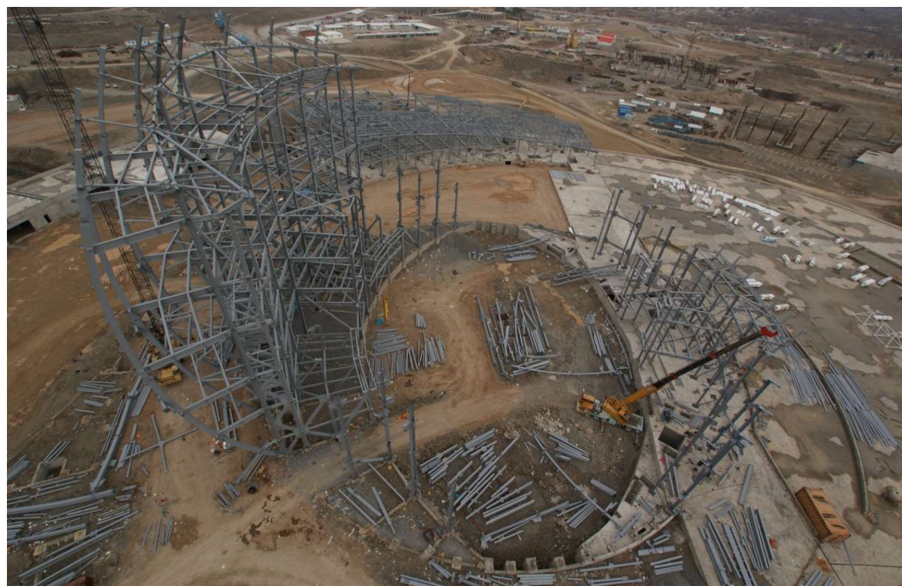
Esfahan International Convention Center, Steel structure of main hall
