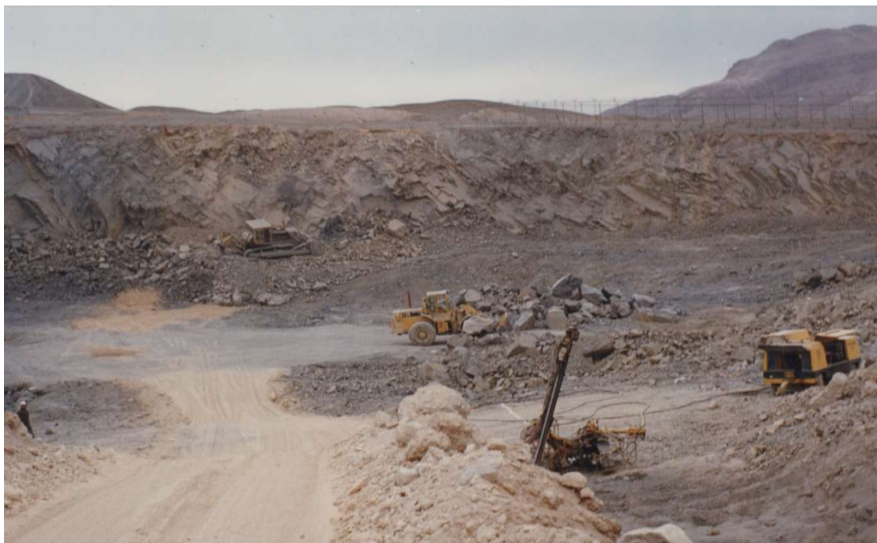
۷۰,۰۰۰ m 3 Water Reservoir in east of Esfahan –Excavation and Rock Cutting
