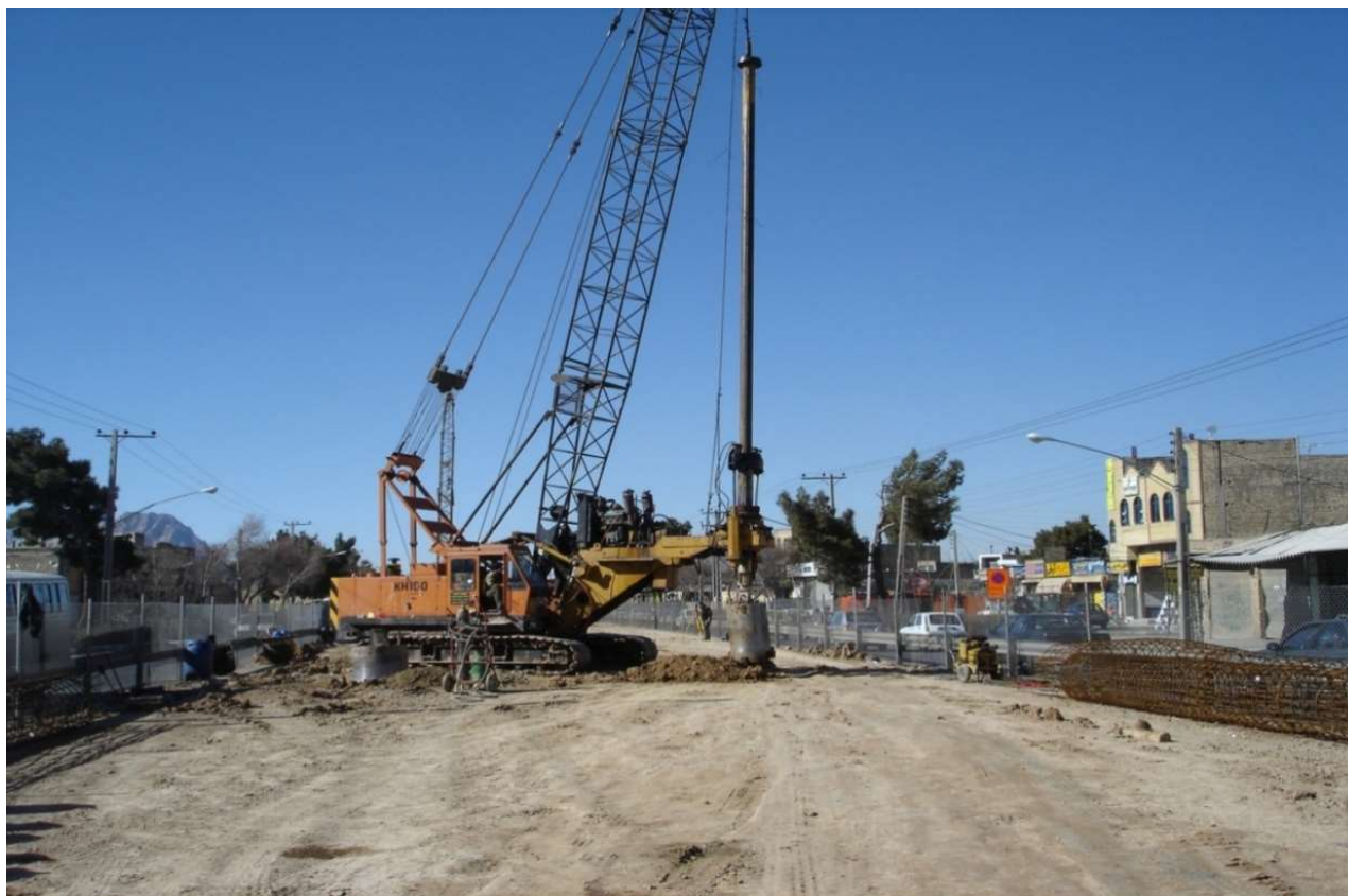
Imam Khomeini highway overpassing bridge, Pilling excavation
