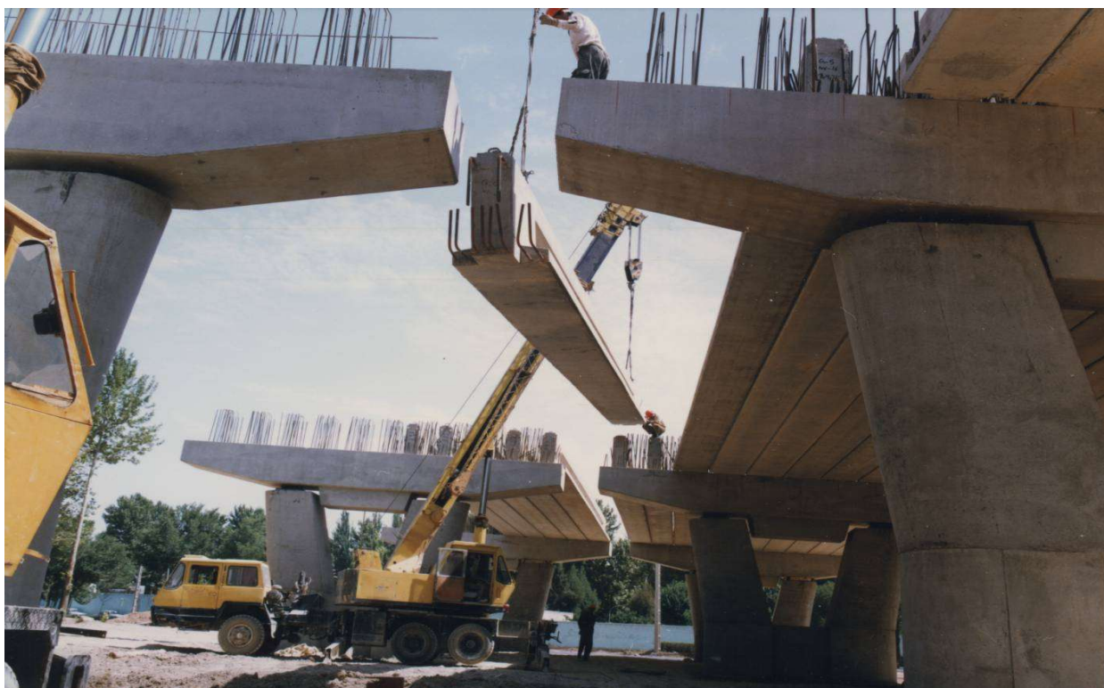
Qadir Bridges complex, Installation of beams and girders
