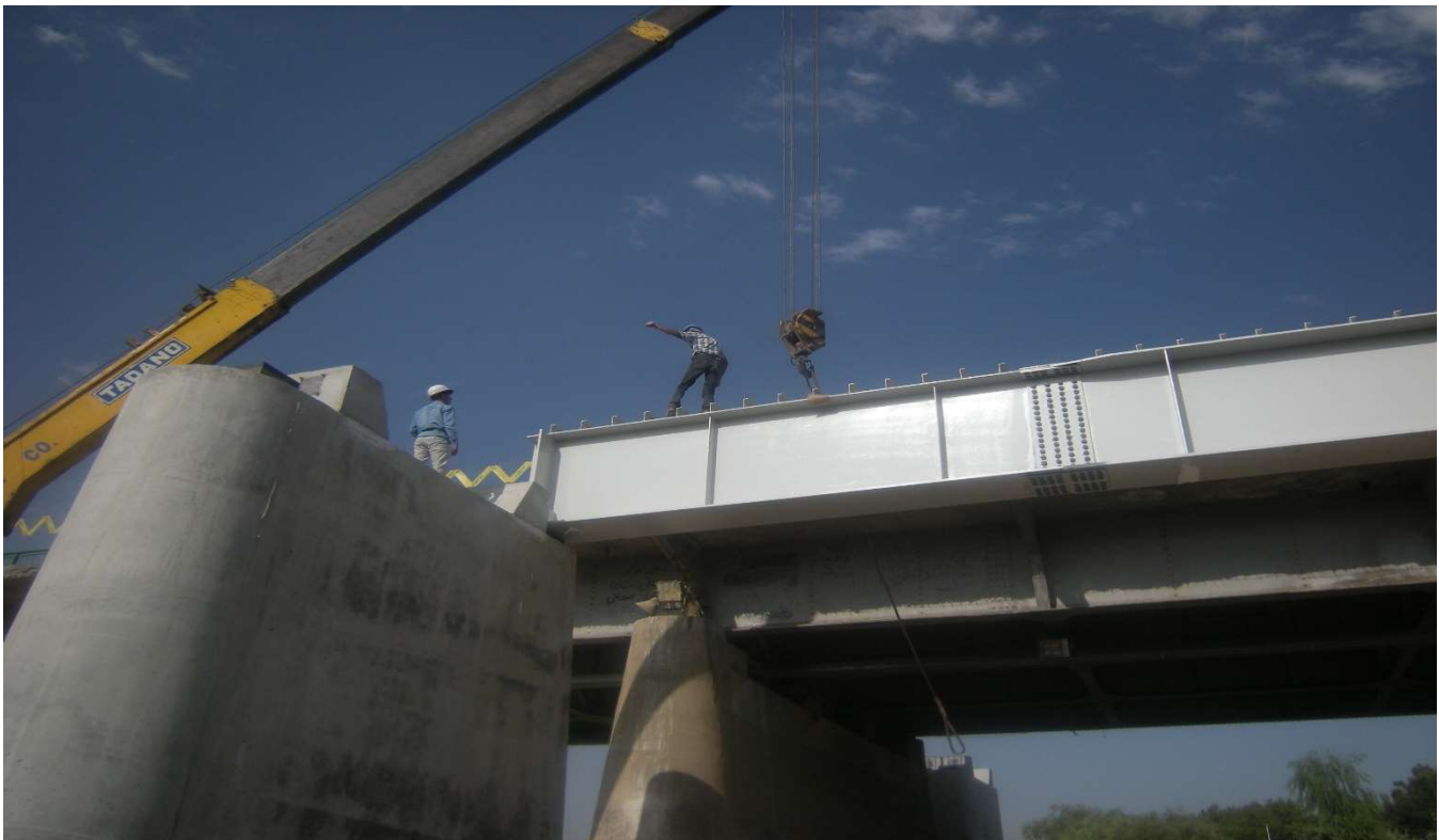
Pol Felezi Bridge, Main Steel Beams Intsallation
