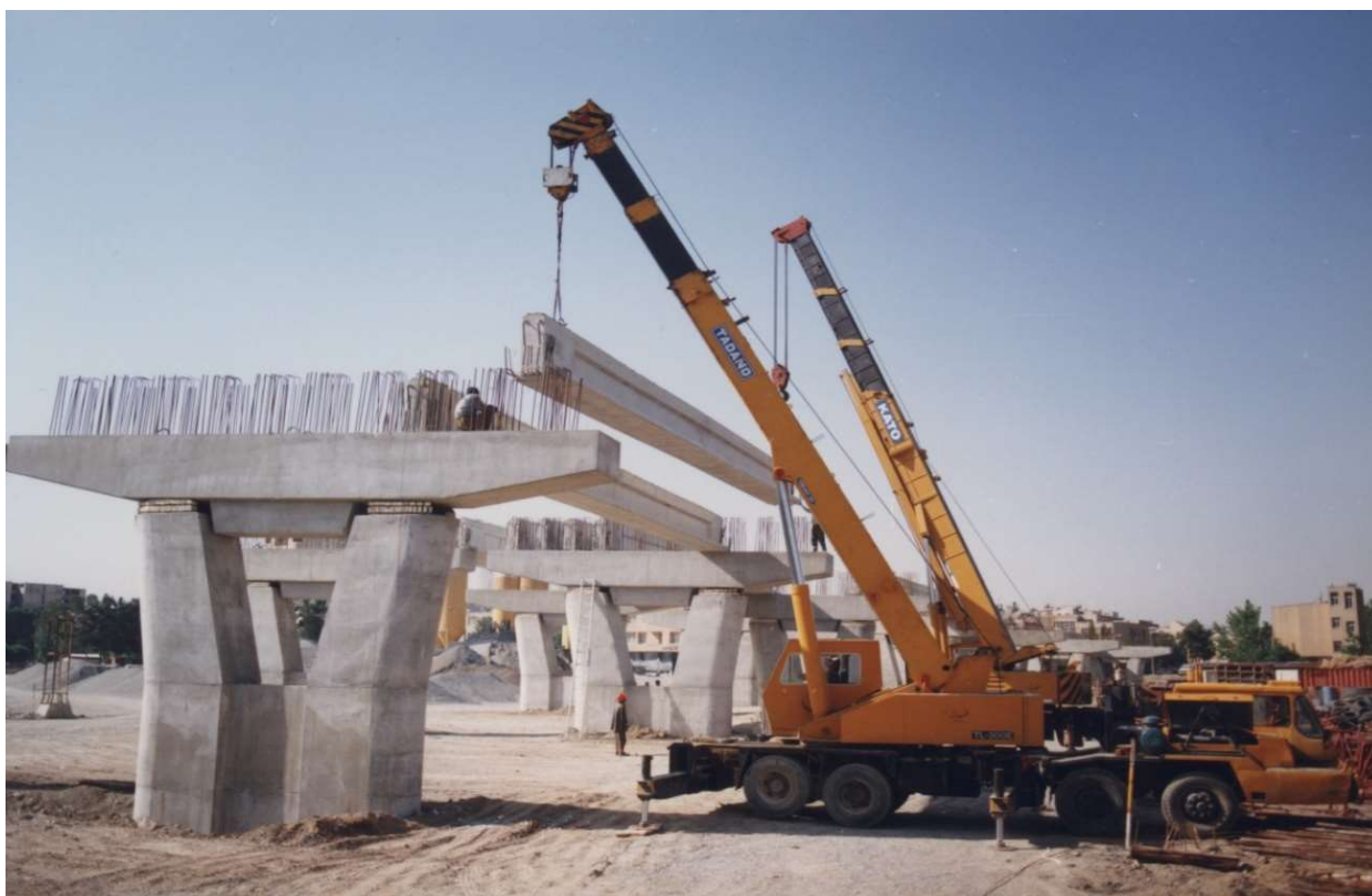
Qadir Bridges complex, Installation of beams and girders
