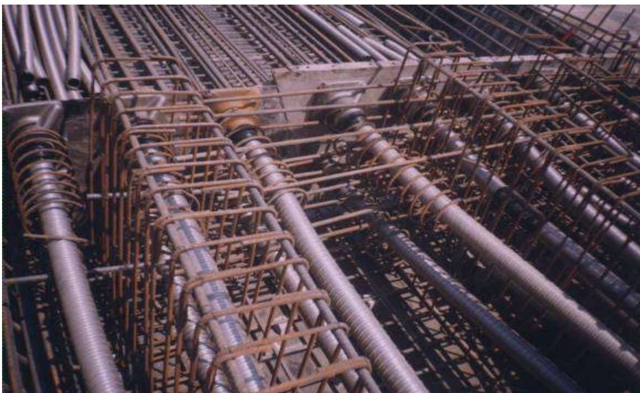
Defea-e-Moqadas Stack Interchange & Flyover, Sleaving of No. 100, 200 and 300 bridge Strands
