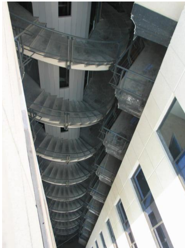
Picture 4 - Nahid Project (Spiral Staircase view from above)
