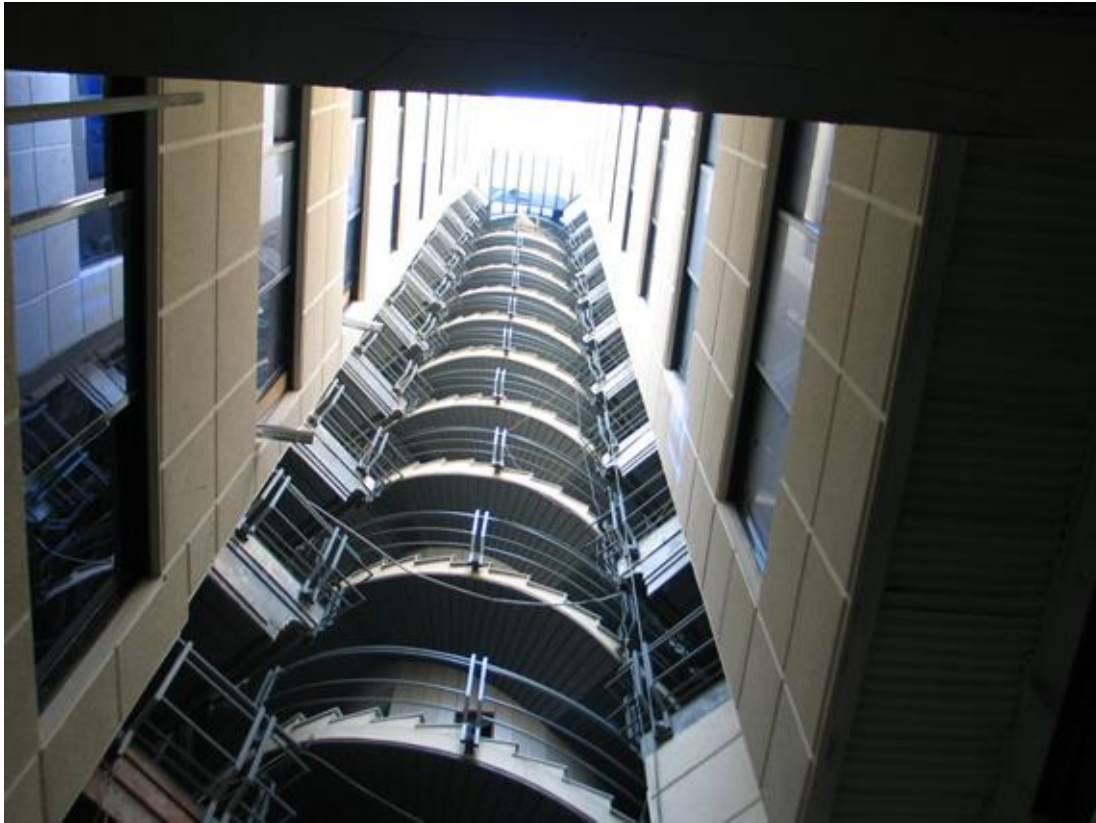
Picture 3 – Nahid Project (Spiral Staircase view from below)
