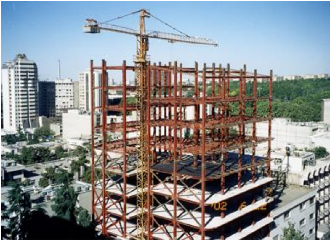
Picture 1 – Nahid Project (Steel Structure Preparation)
