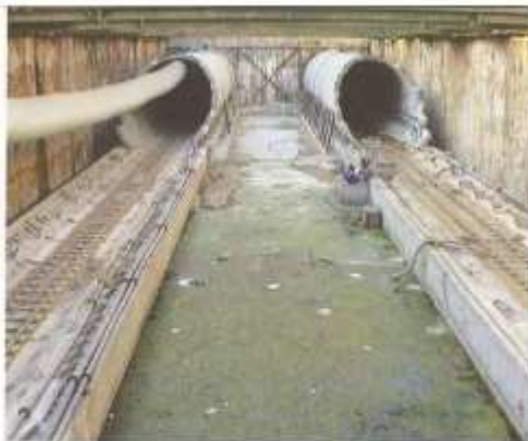
Concrete TBM cradles
