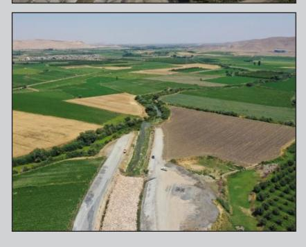
THIS PROJECT INCLUDES A TRAPEZOI-DAL CANAL WITH CONCRETE COVER AND MASSIVE CONCRETE STRUCTURES, WHICH INCLUDES THE FOLLOWING TWO MAIN PARTS:
